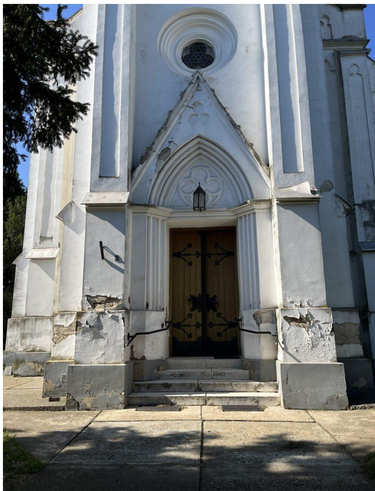
Figure 6: The Church of the Exaltation of the Holy Cross – Saint Eleanor in Tiszavasvári in its pre-renovation condition 21
